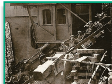
Workers constructing the Cambria Incline
