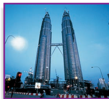
Petronas Tower I
